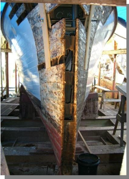
Caretaking of a classic wooden boat to keep it healthy is a constant task. Olmaha has had electrical system updating, mechanical maintenance, annual bottom painting, periodic hull and brightwork re-finishing, as well as caulking, refastening and occasional new planking. In addition she has also presented some larger shipwright challenges for "big timber" items. Here is a little photo essay of three of these.
