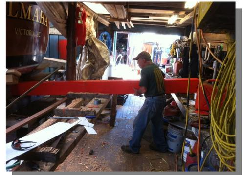
The new timber was coaxed in over the deadwood and new bolt tops were driven down the pre-bored holes and welded to the old bolt stubs protruding from the deadwood. The new horn timber was then dogged down onto the deadwood and a new transom knee was fitted over the old bolts in the transom, keeping it undisturbed.
